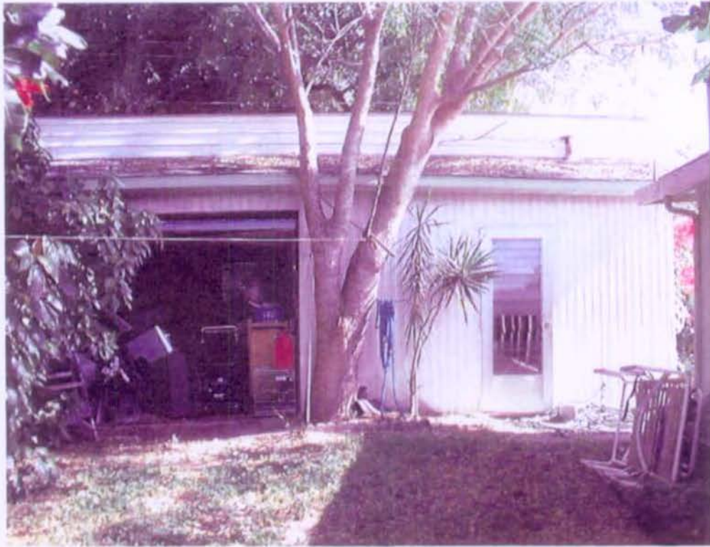
VIEW LOOKING EAST FROM DRIVEWAY TOWARDS GARAGE / STORAGE BLDG.
