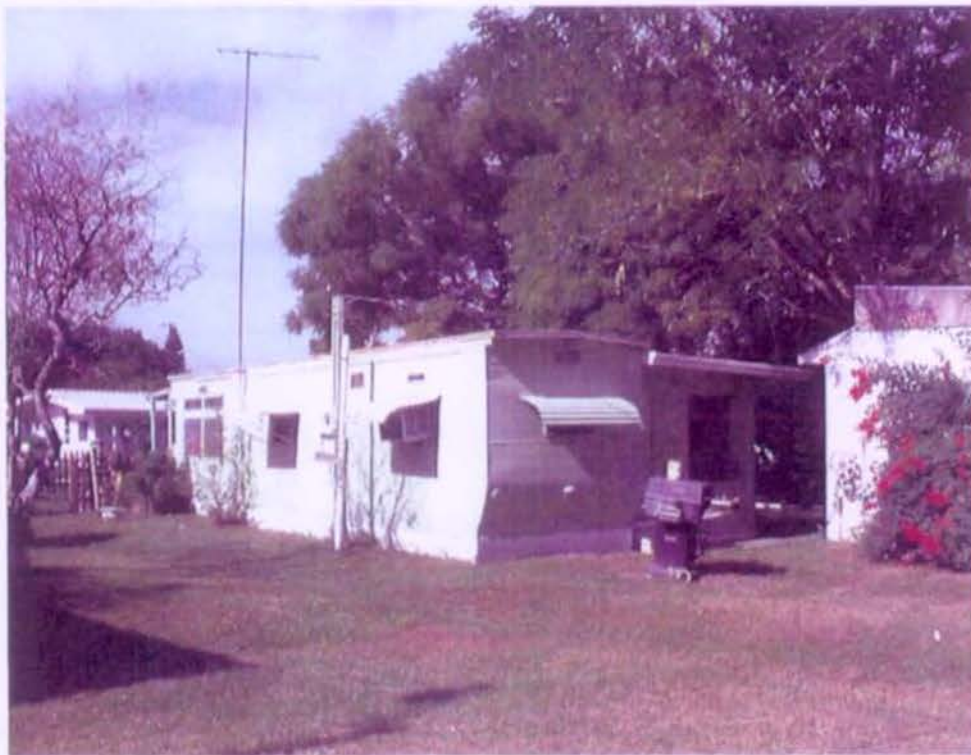
VIEW LOOKING NW FROM SW CORNER OF PROPERTY, TOWARDS REAR OF RESIDENCE
