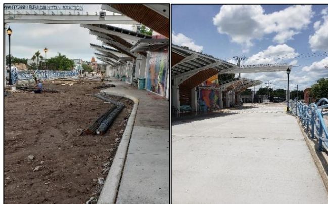
2020 Downtown Transfer Station Upgrades: Before and After
