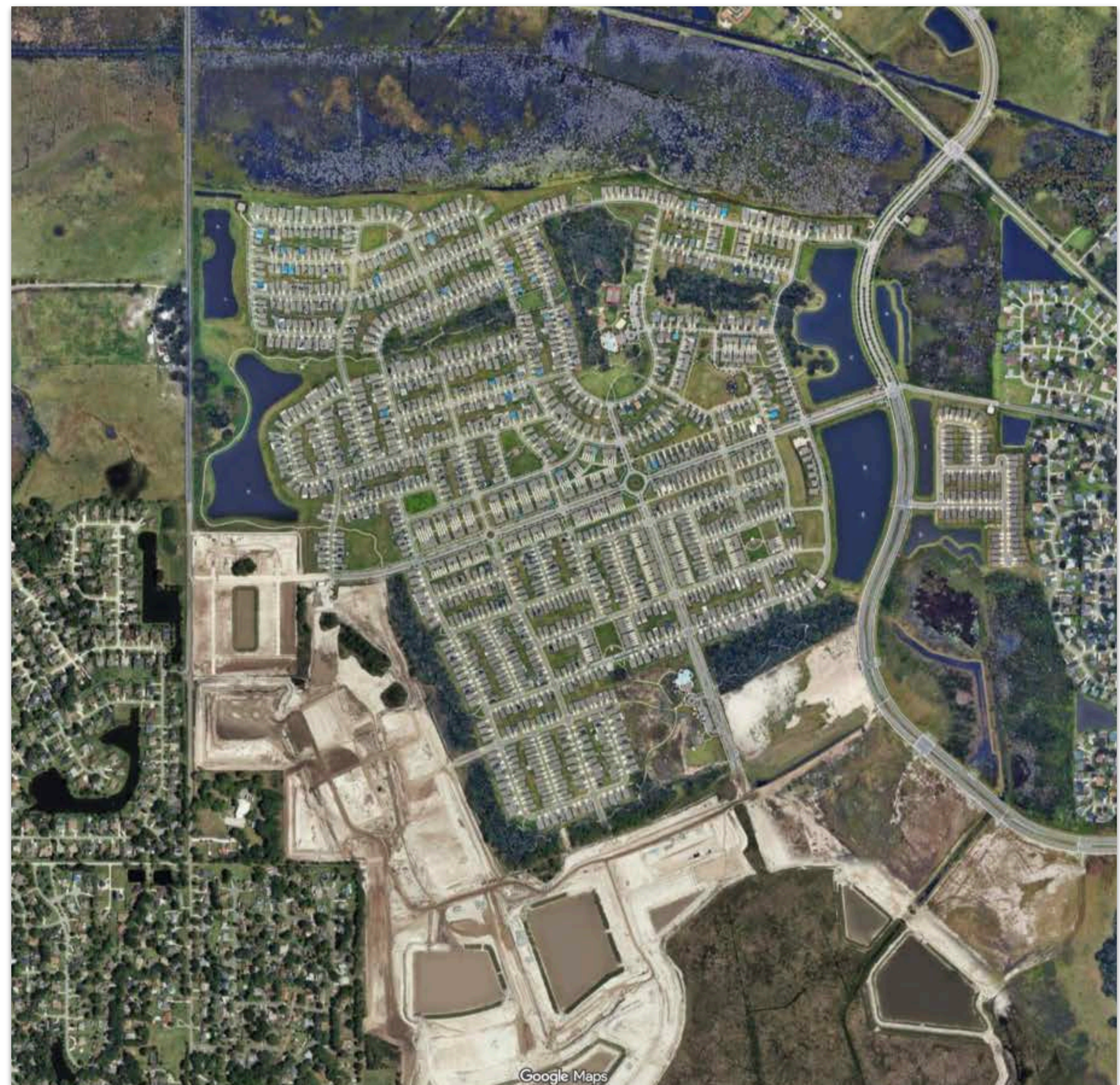
Portion of completed development. Image Credit: Google Maps
