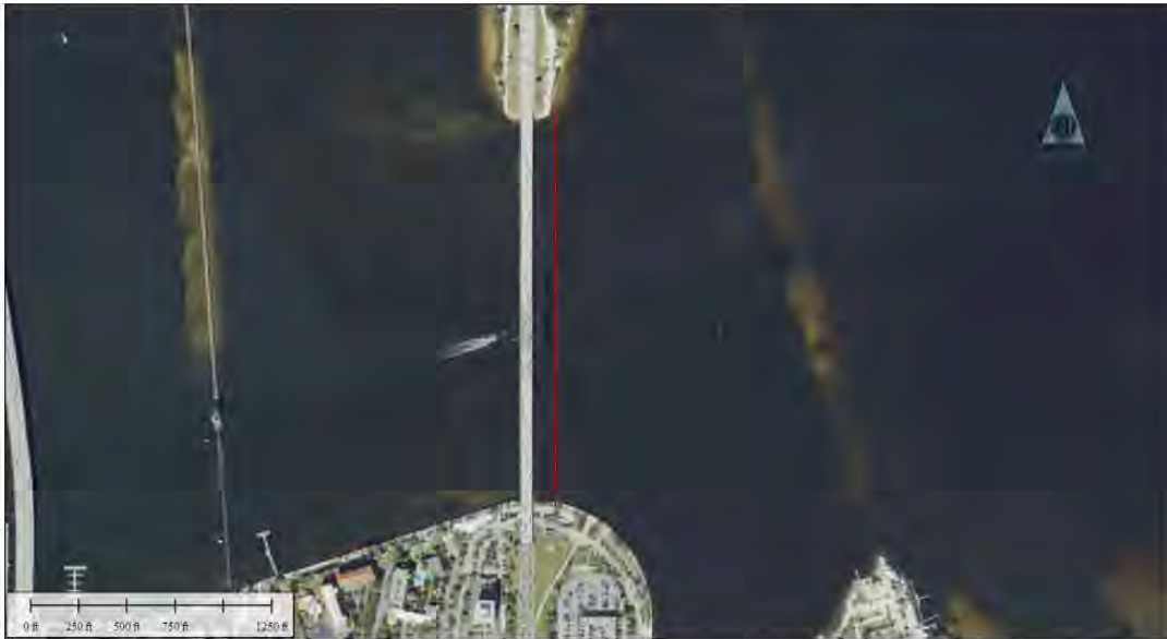
Figure 3: The pipeline (shown as a red line) crossing at the Desoto Bridge is subaqueous for the entire length and is located 150 ft east of the bridge centerline.
