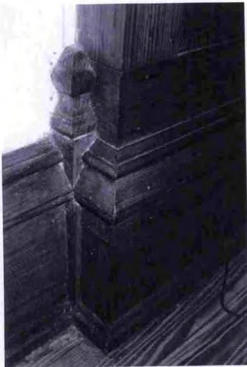
PHOTO 20, Detail of corner baseboard next to living room opening column base, looking southeast
