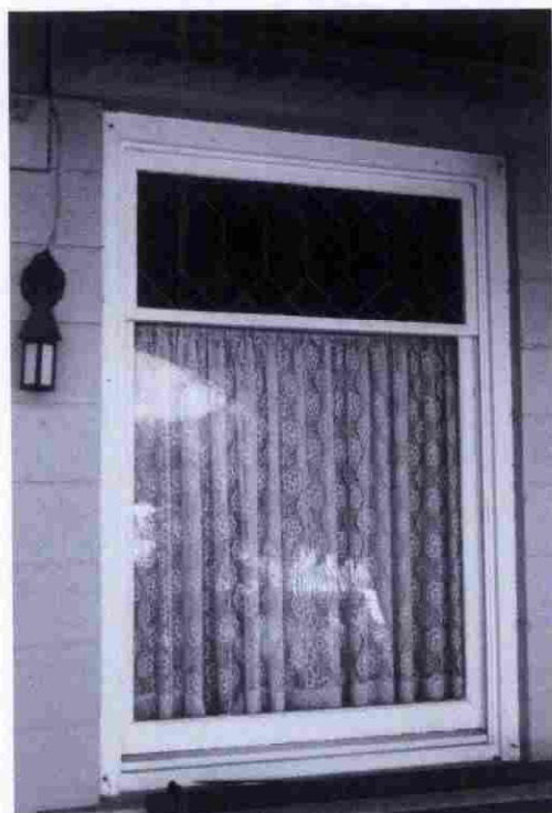
PHOTO 4, Detail view of foyer window showing leaded glass in top pane, looking southwest
