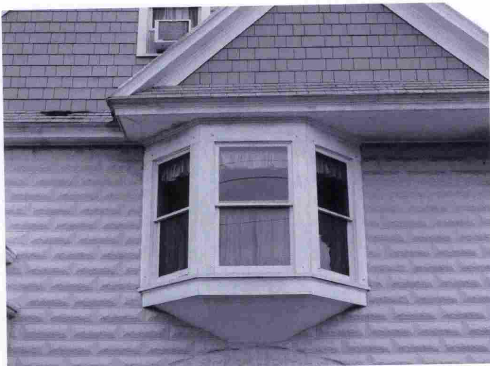
PHOTO 5, Detail view of oriel window, looking south
