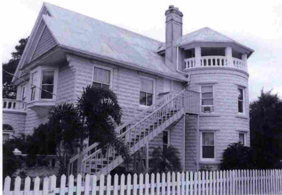
PHOTO 12, West and north elevations, looking southeast
