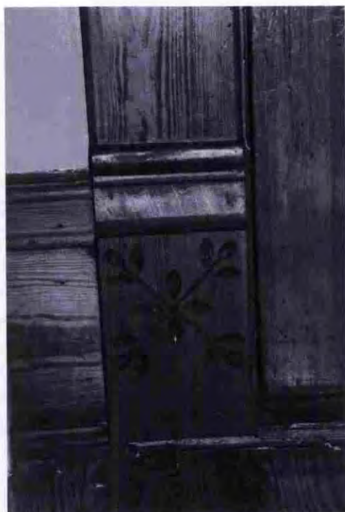
PHOTO 23, Detail of carvings within kitchen baseboard
