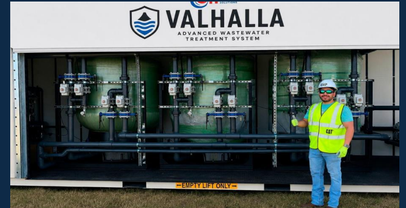
CHC / treatment — interior
