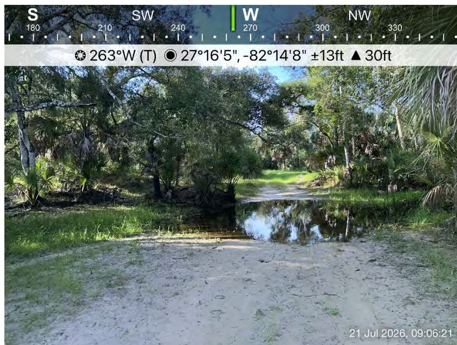
Photo 8: Low water crossing observed on the Subject Property.
