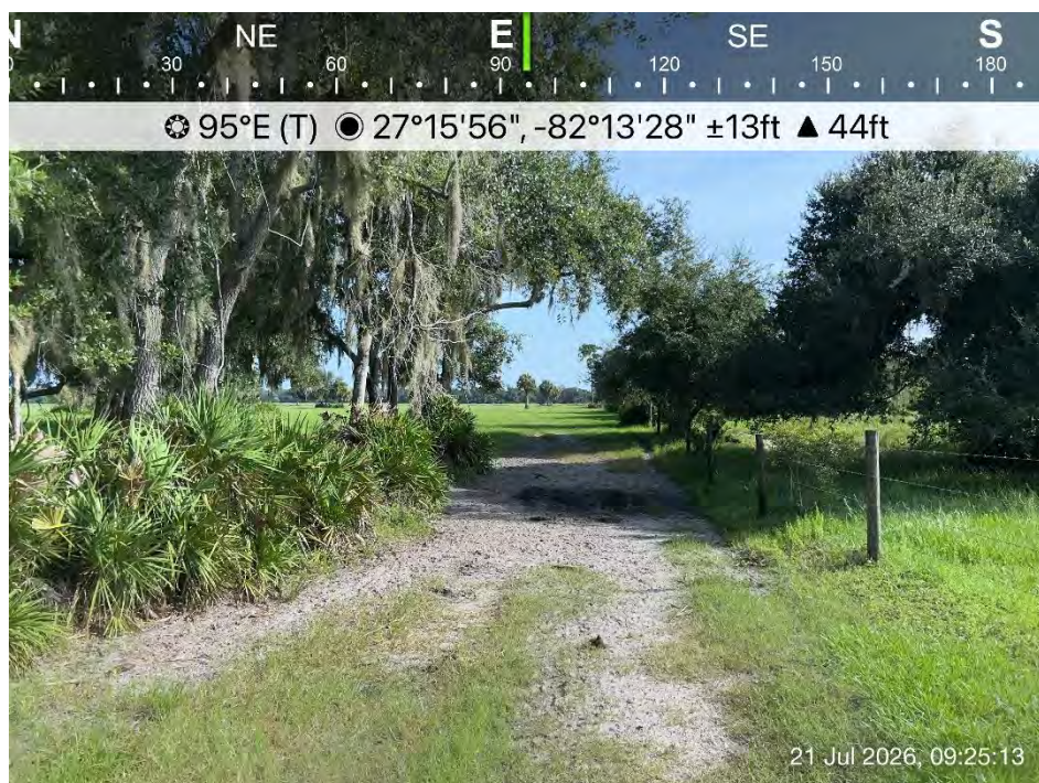
Photo 18: Overview of low water crossing and Subject Property.
