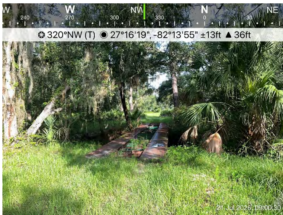
Photo 5: Bridge observed on the Subject Property.
