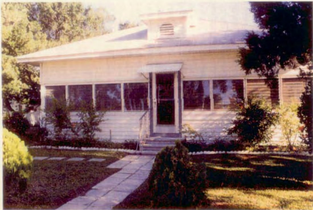
Residence to detached garage
