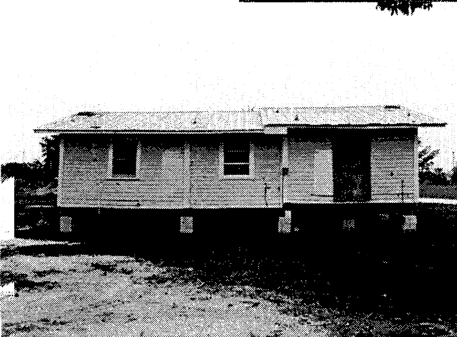
Blue House 302 Bay Drive South to 4524 123rd Street West
