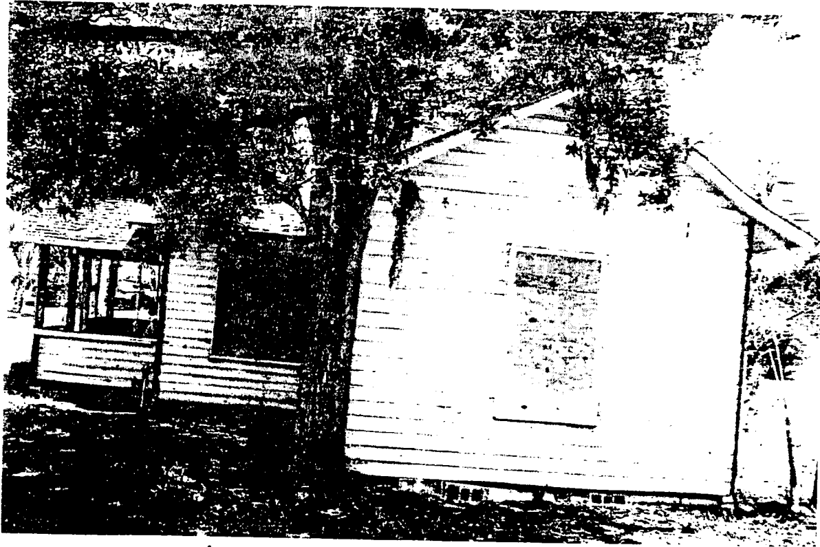
SUBJECT WEST SIDE
