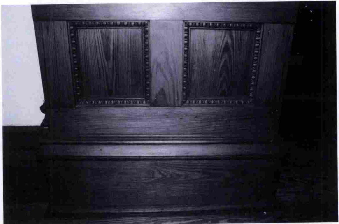
PHOTO 19, Detail of living room opening column base, looking east
