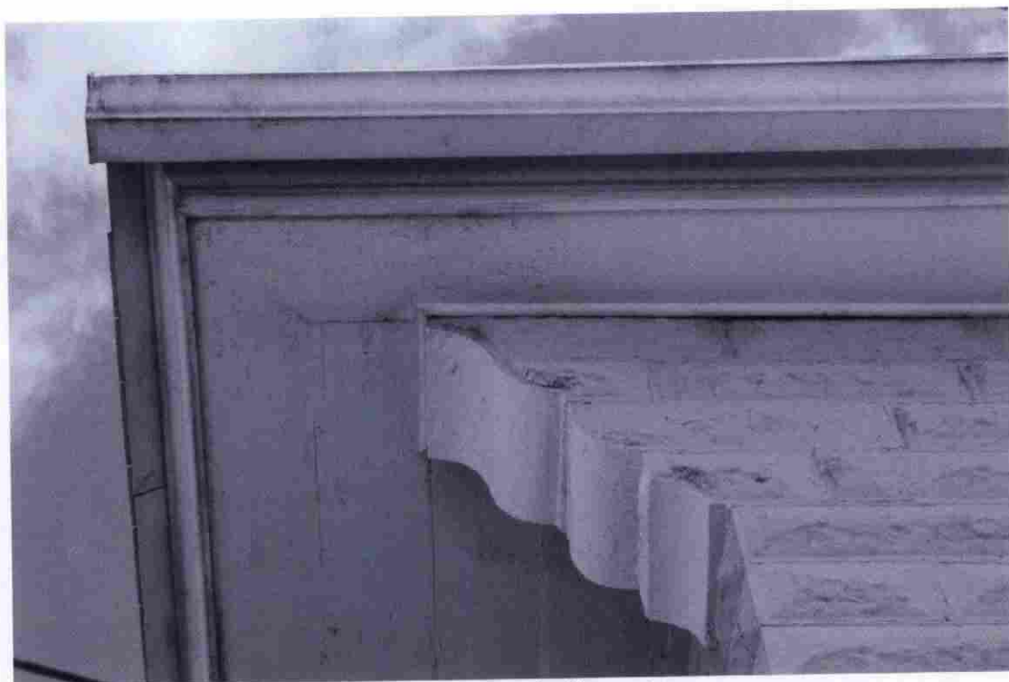
PHOTO 6, Detail of corner bracket at northwest corner, looking east
