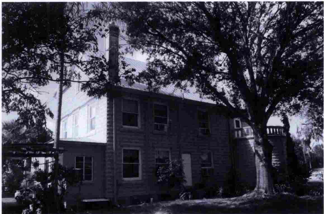
PHOTO 10, East elevation, looking northwest
