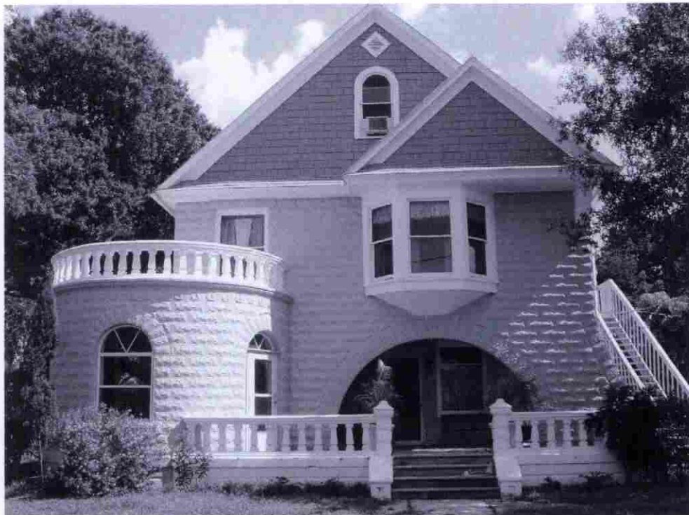
PHOTO 2, North elevation, looking south
