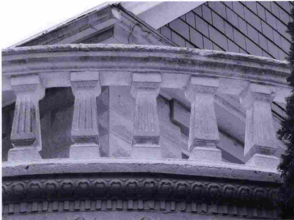
PHOTO 9, Detail view of balustrade on northeast roof terrace, looking southwest
