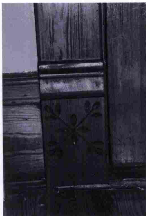
PHOTO 23, Detail of carvings within kitchen baseboard
