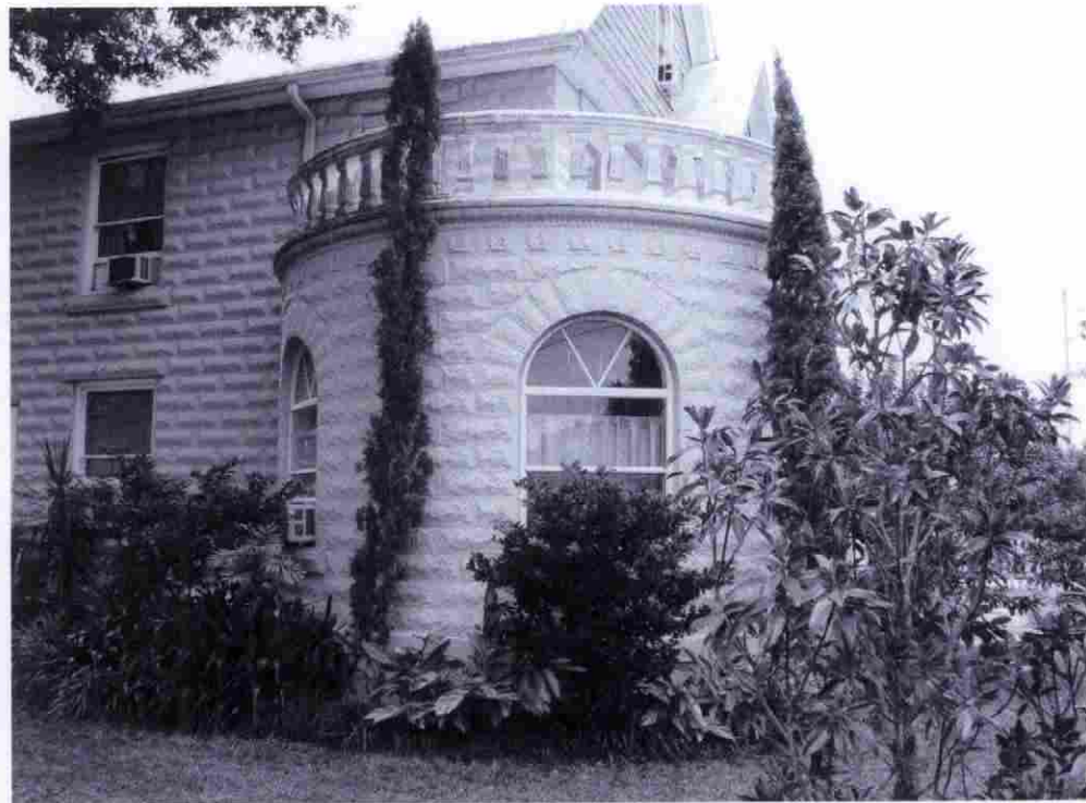
PHOTO 8, Detail view of northeast tower, looking southwest
