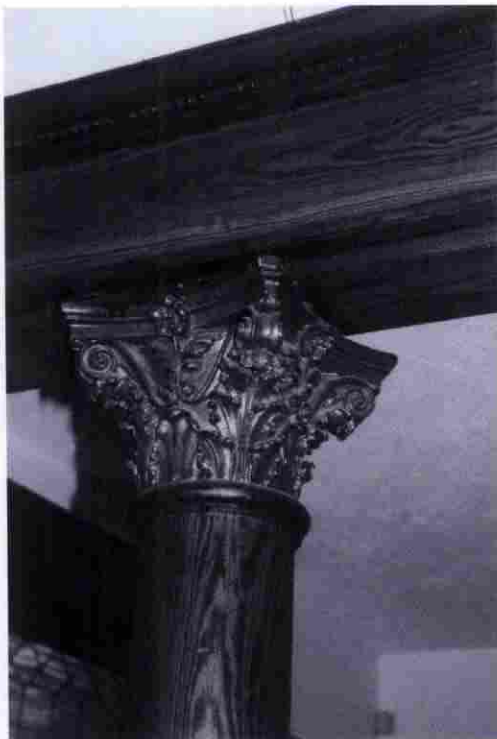
PHOTO 18, Detail of capital on living room opening columns, looking northeast
