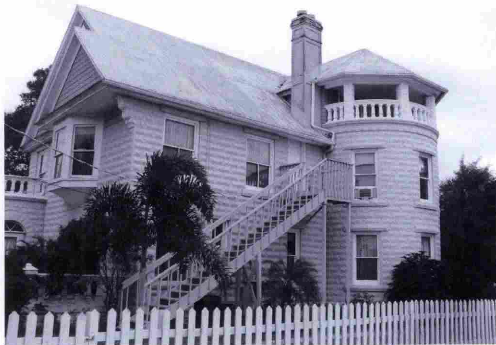
PHOTO 12, West and north elevations, looking southeast
