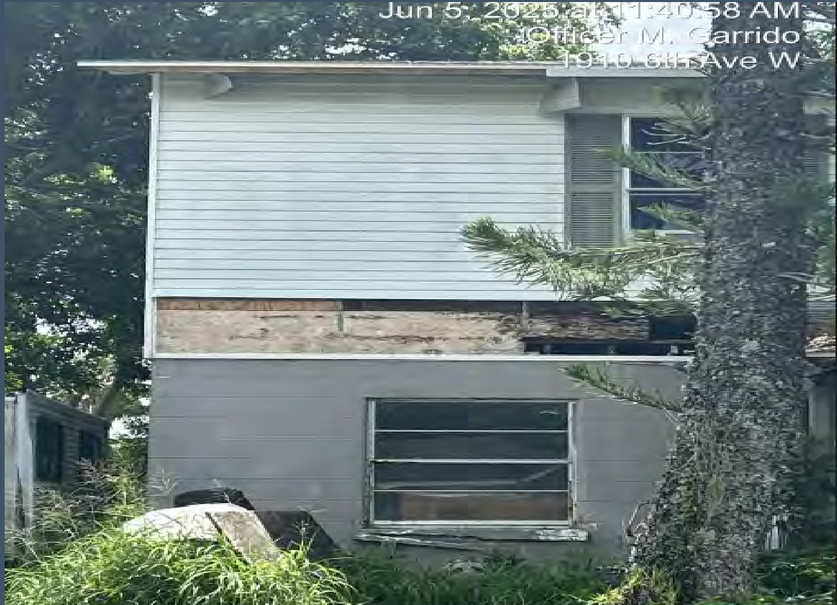
View of the front side of the property.
