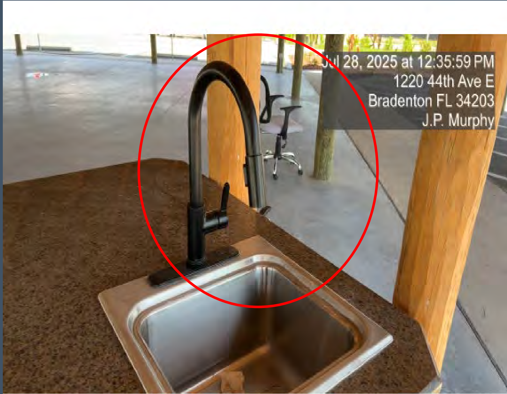
View of the plumbing from the property.
