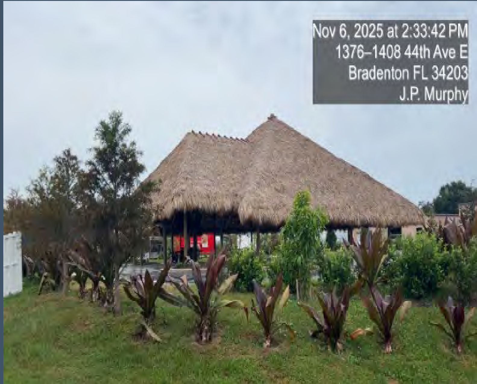
View of the structure from 44 th Ave E.
