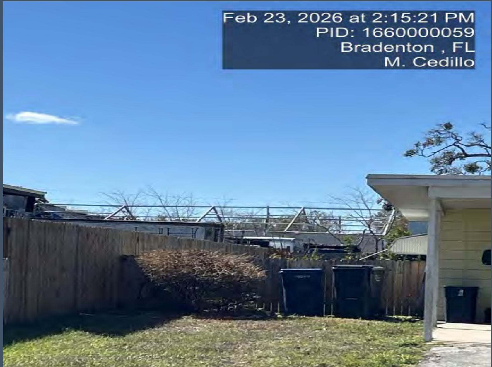
View from the street of the unpermitted structure
