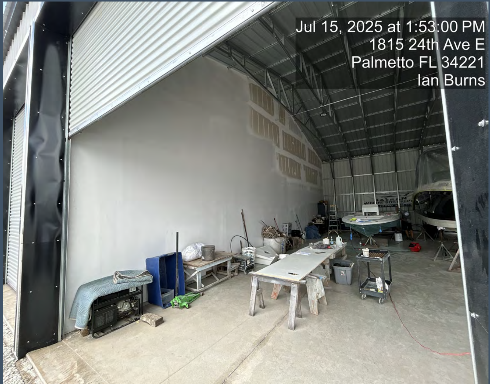
Photo depicts the interior walls that were installed
