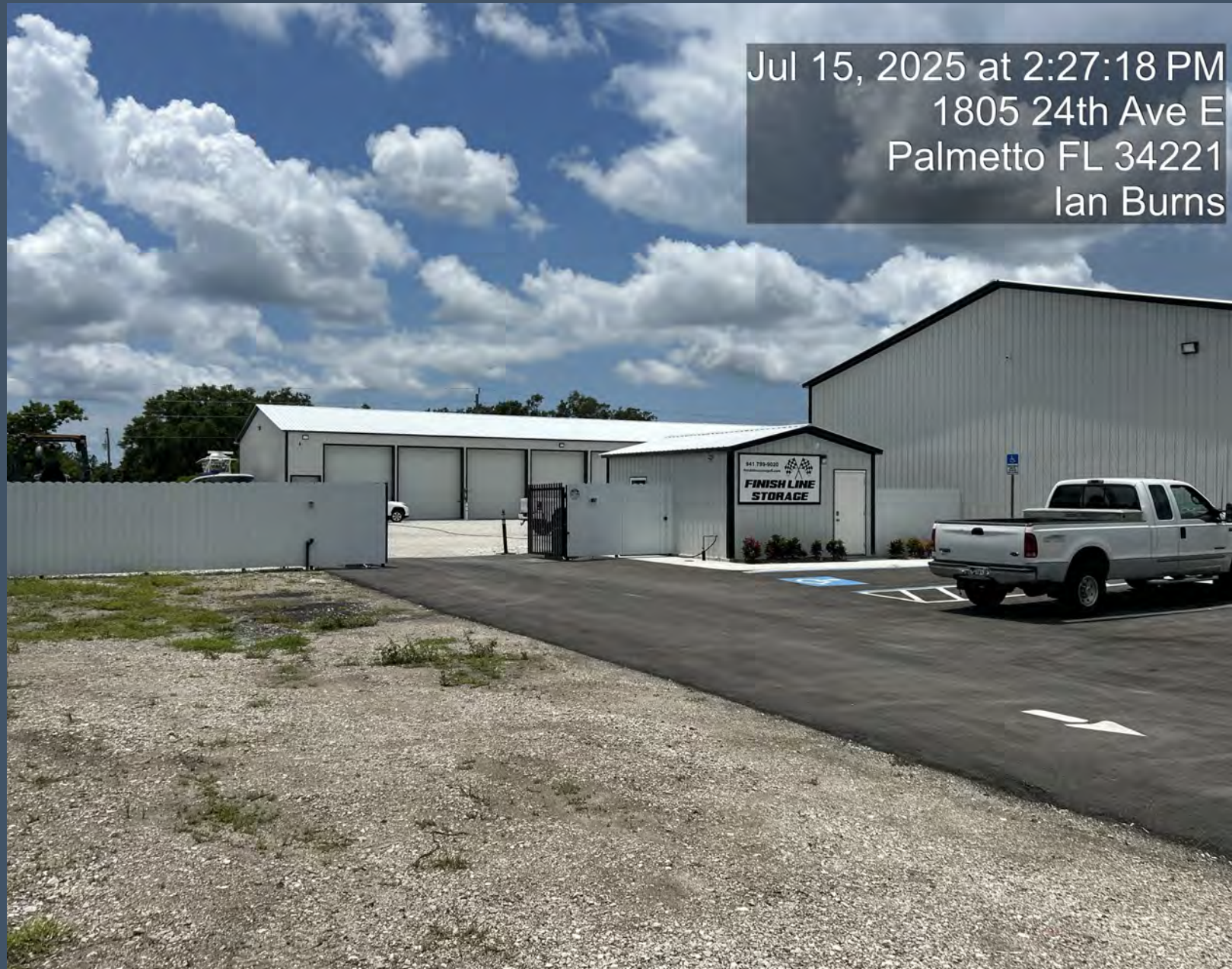
Photo depicts the front of the property
