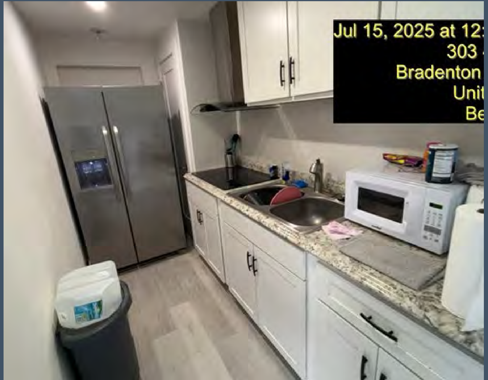
View of rear unit renovations.
