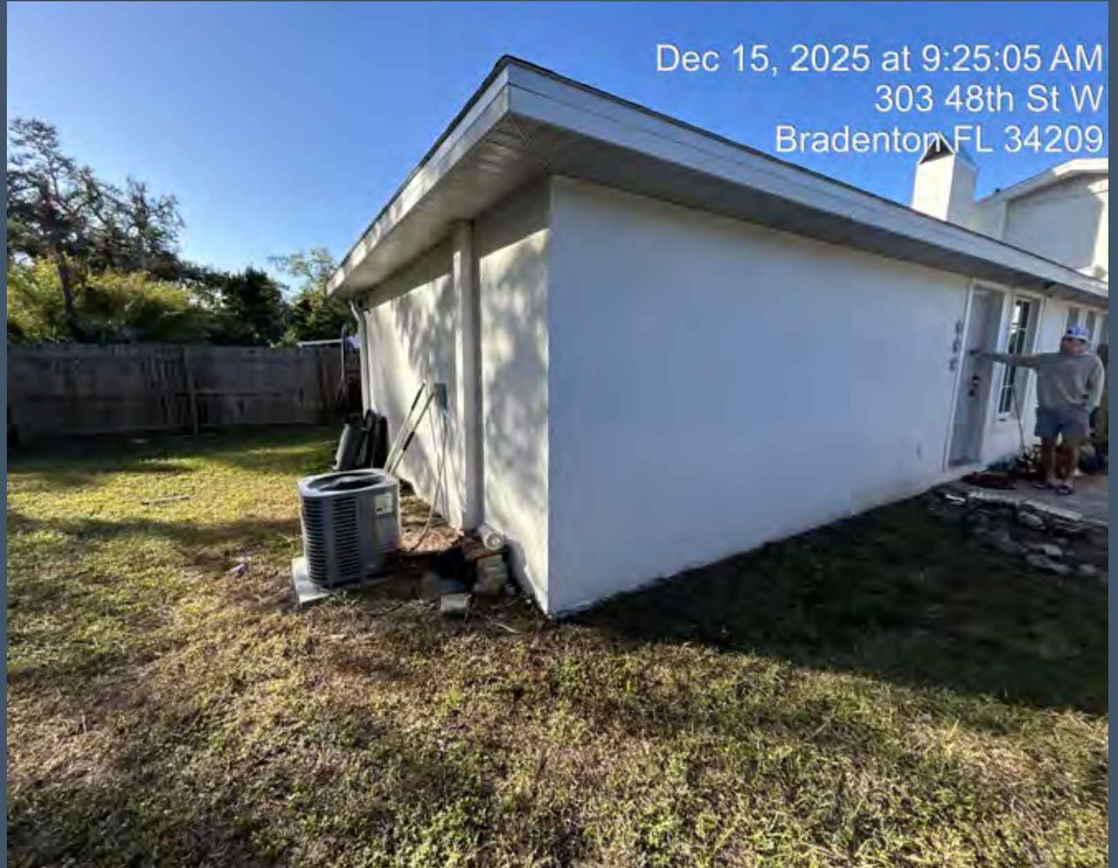
View of the rear of the structure.
