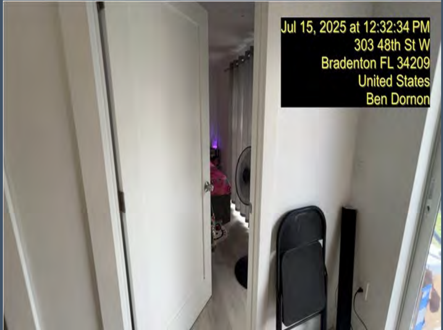
View of rear interior wall for second bedroom.
