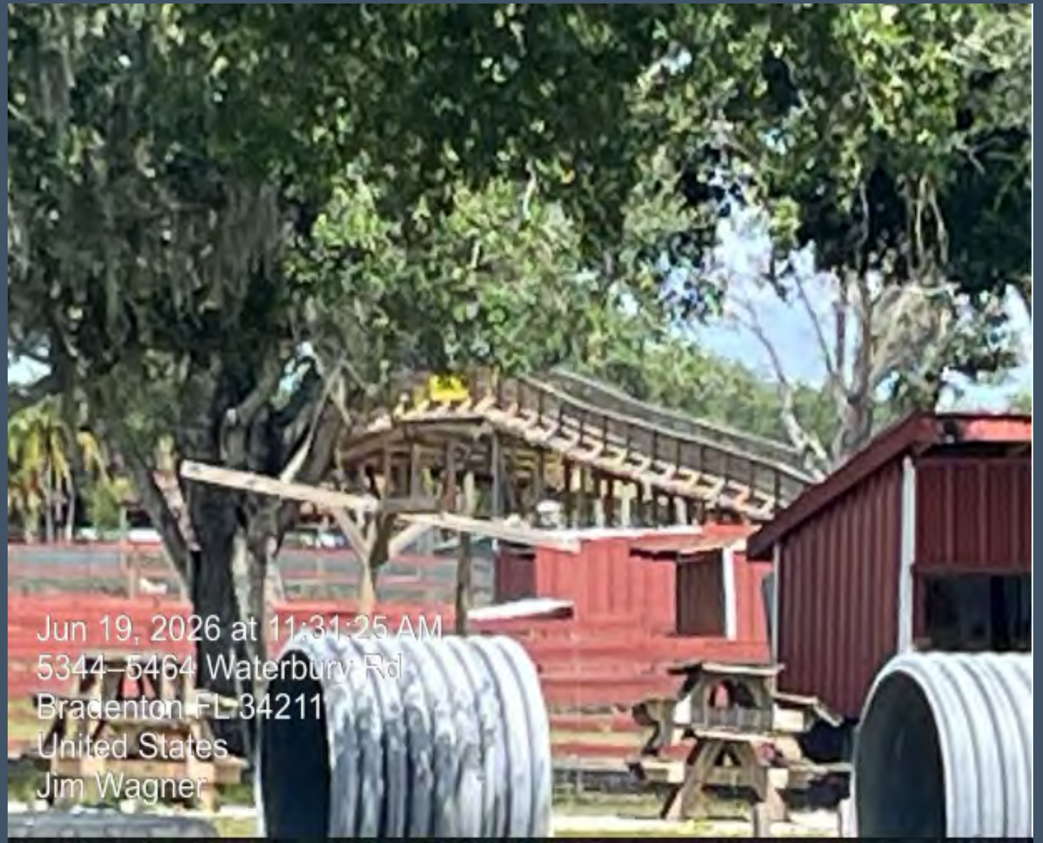
View of the bridge from the road.
