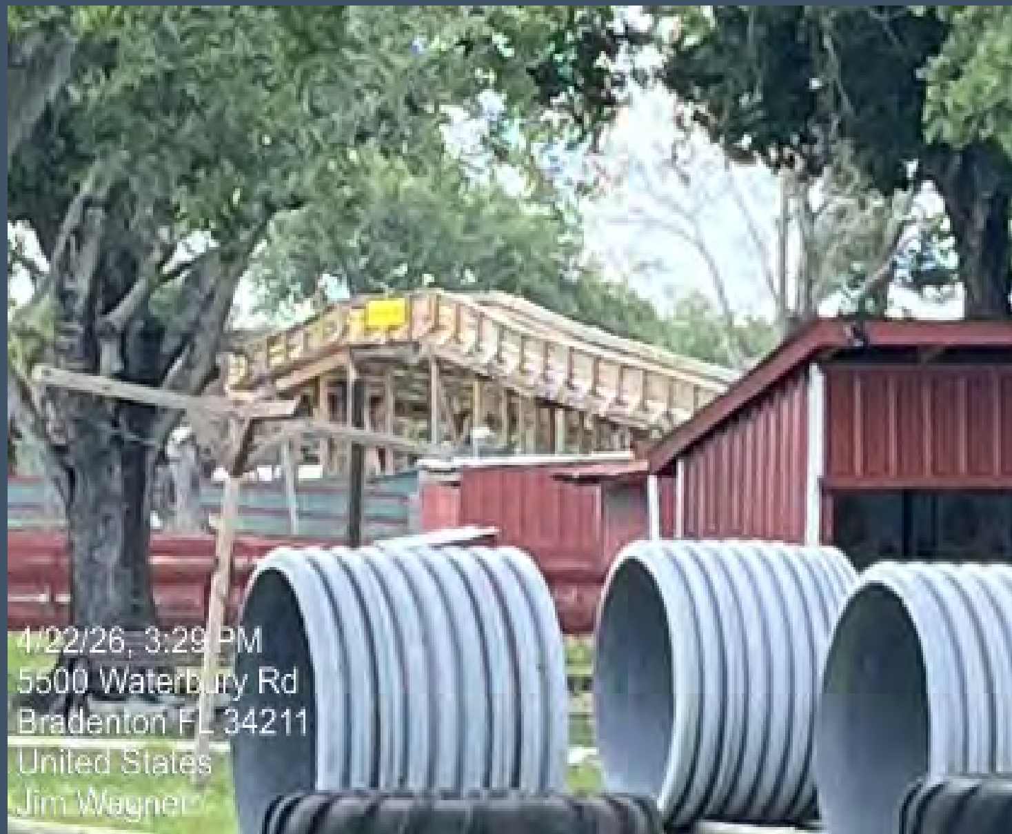
View of the bridge from the road.
