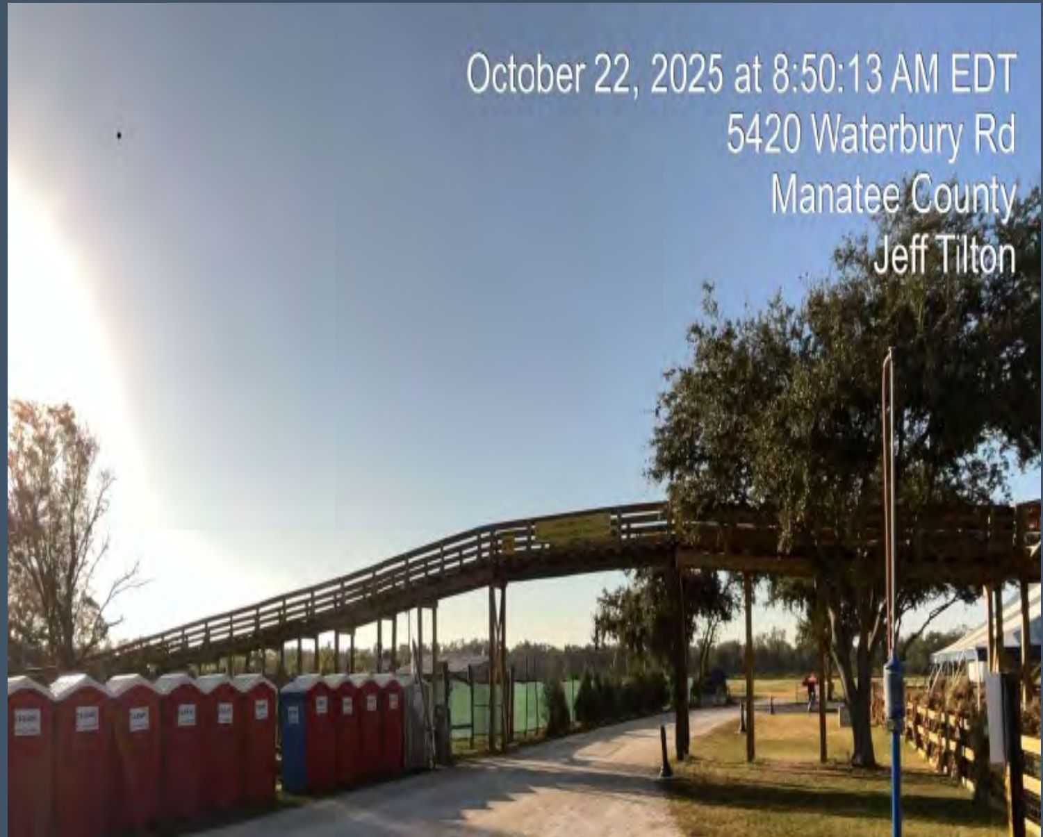
View of the bridge from the property.
