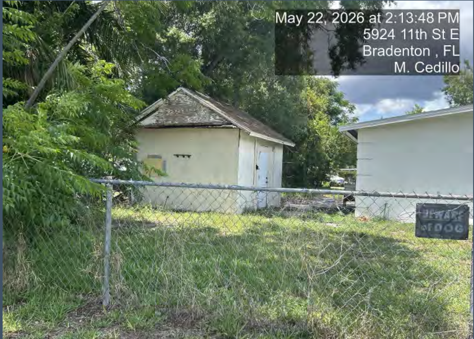
View from street of the unpermitted structure
