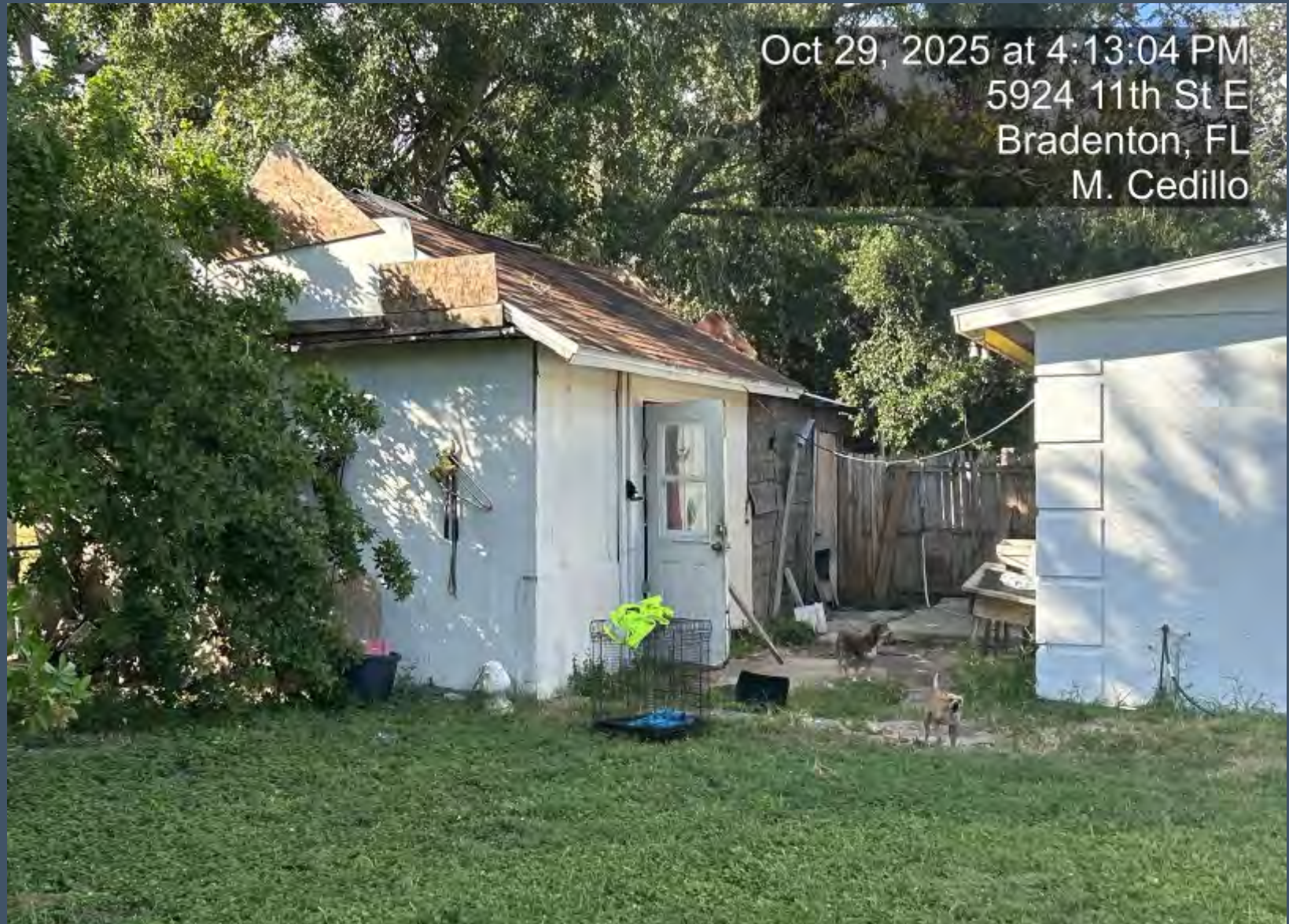
View from street of the unpermitted structure
