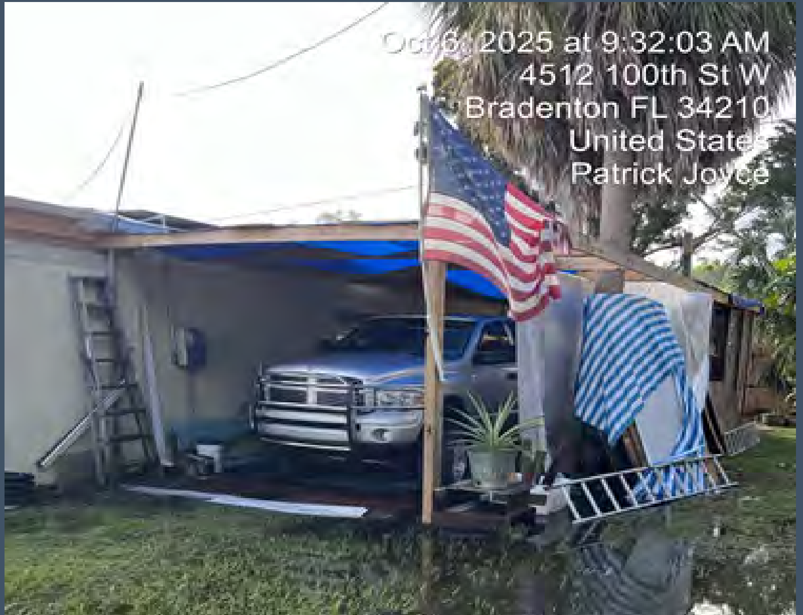
Photo of the unpermitted carport attached to the unpermitted pole barn
