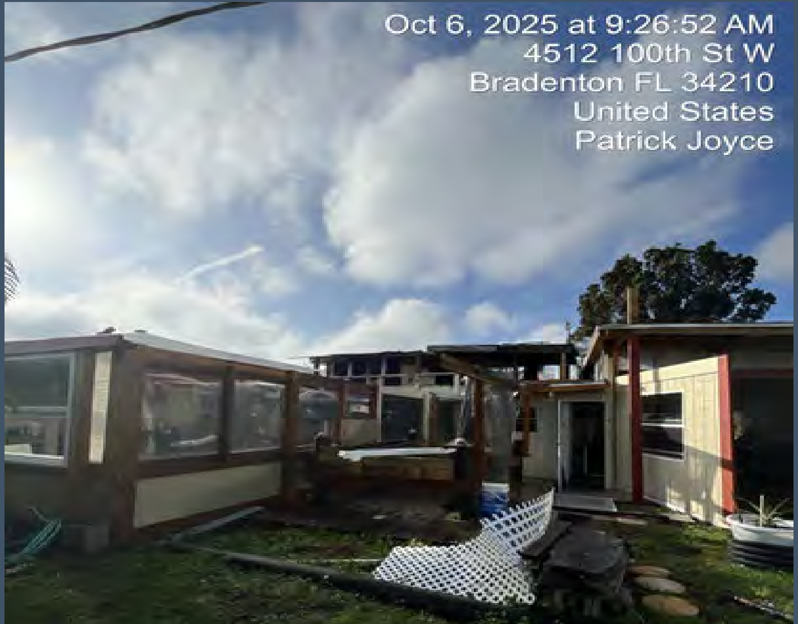
Photo of an unpermitted deck, pool cage, and pole barn
