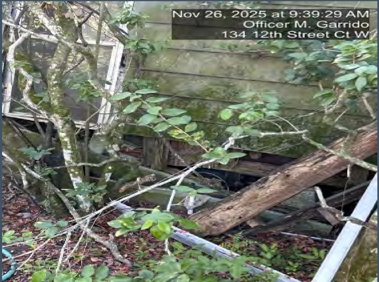
View of the north (rear) wall of the property.
