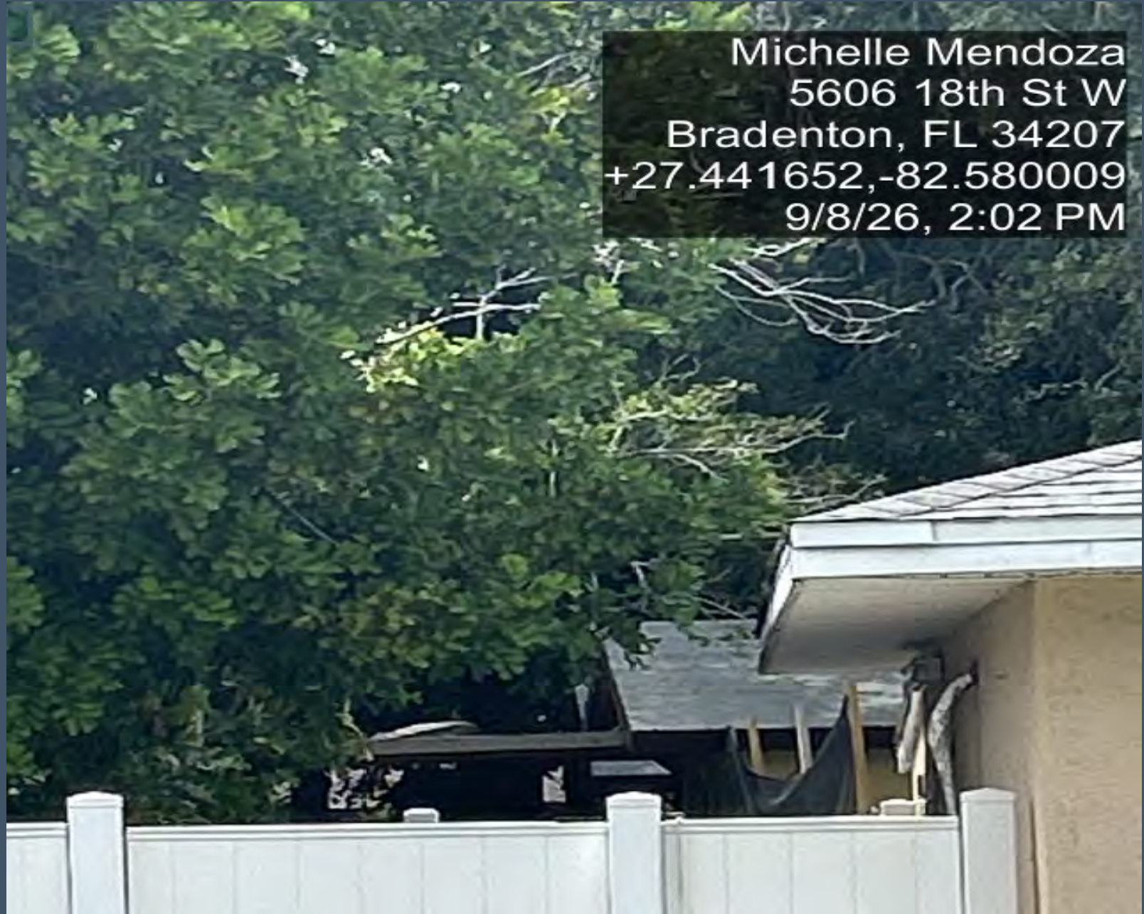
Photo of the structures still present.
