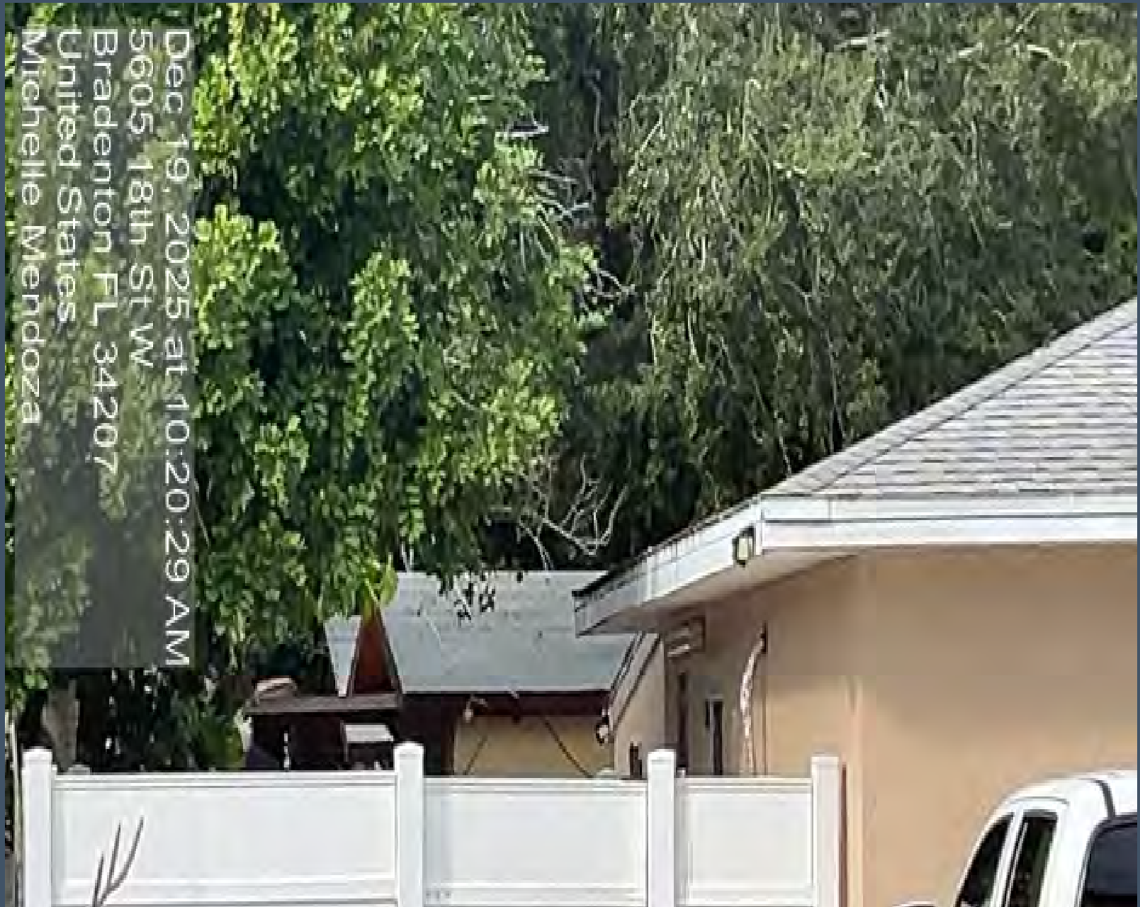
Photo of both structures from the front of the property.
