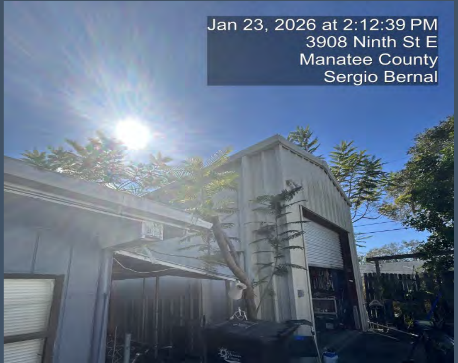
Photo of the unpermitted shed located in the rear of the property (01-23-2026)
