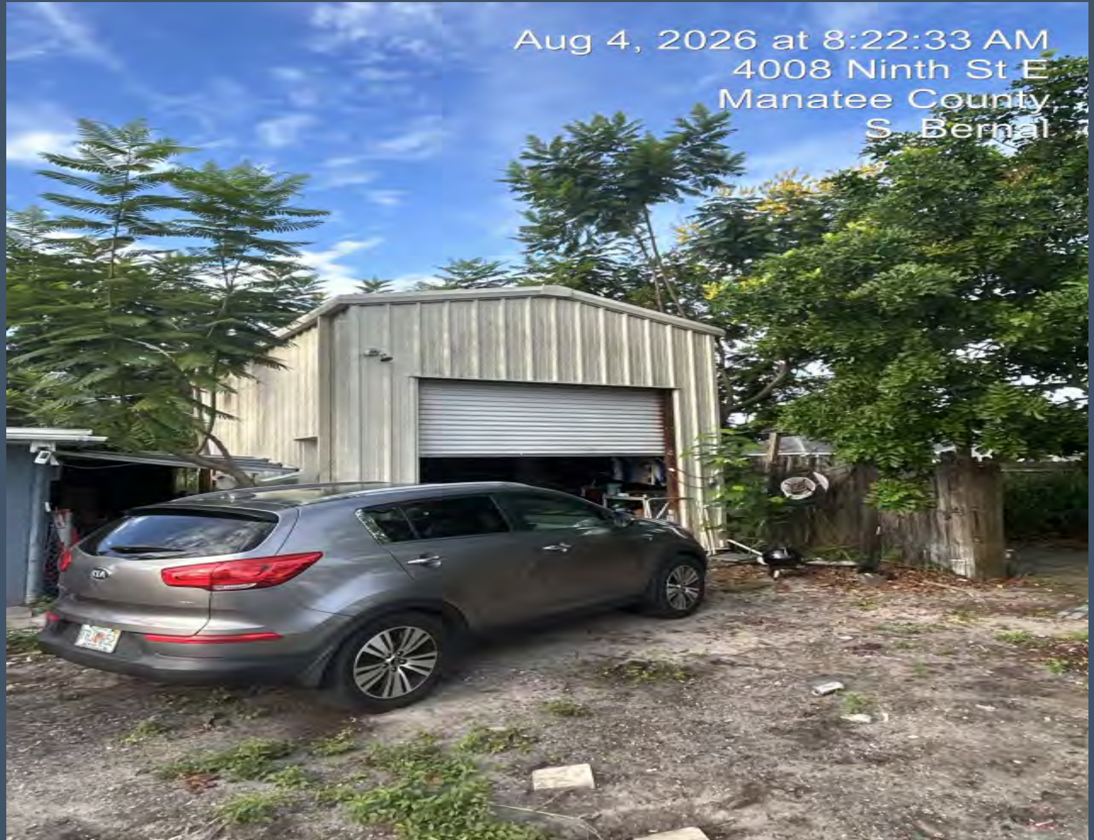
Photo of the unpermitted shed located in the rear of the property.(08-04-2026)
