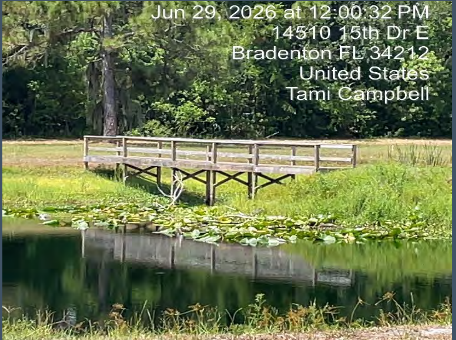
Bridge built across the pond
