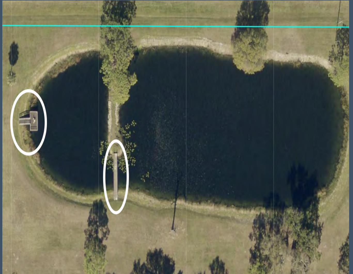
Aerials of dock and bridge built on pond
