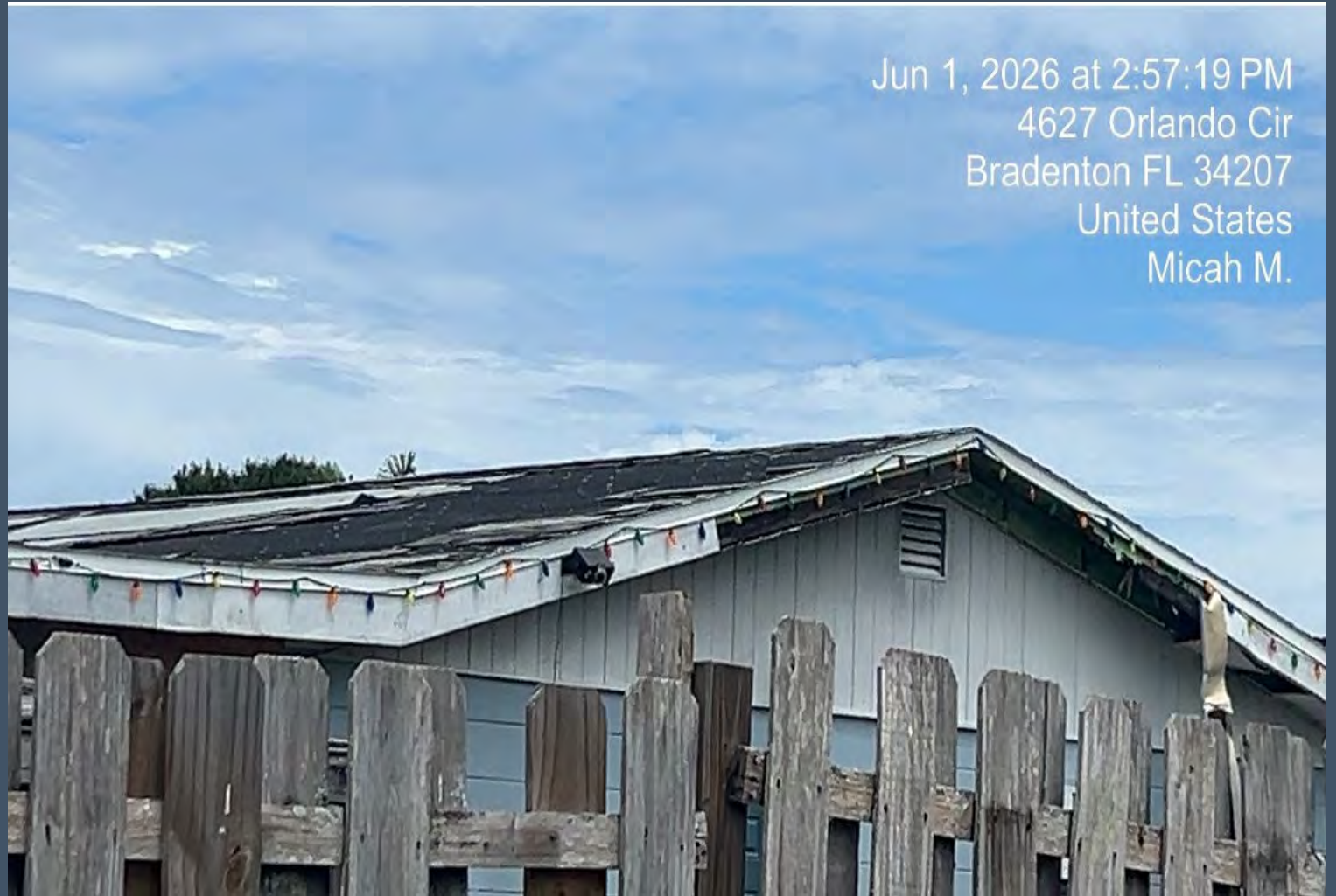
REAR VIEW OF ROOF FROM THE STREET
