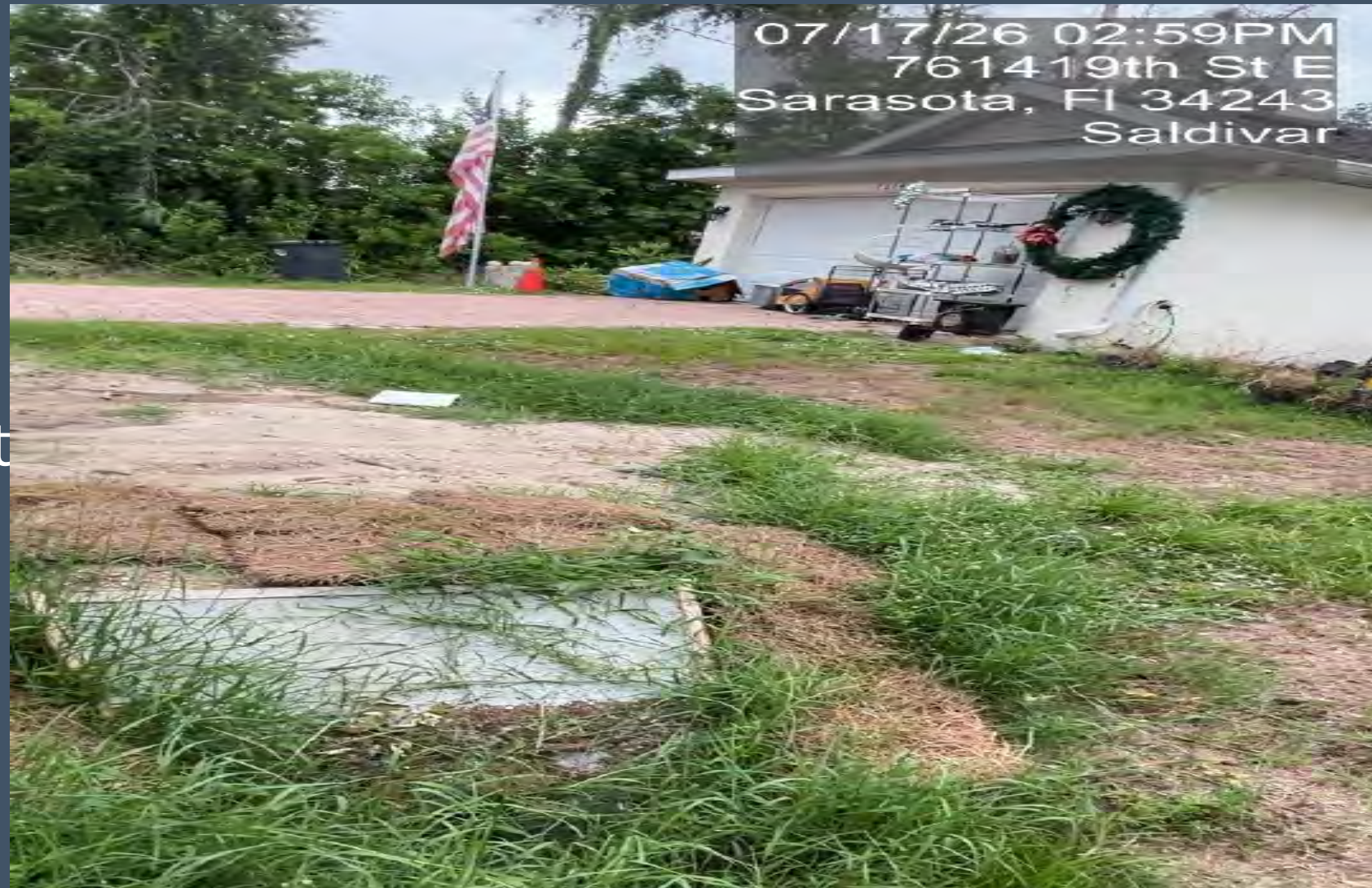
Picture depicts the culvert (with concrete) still on the property.
