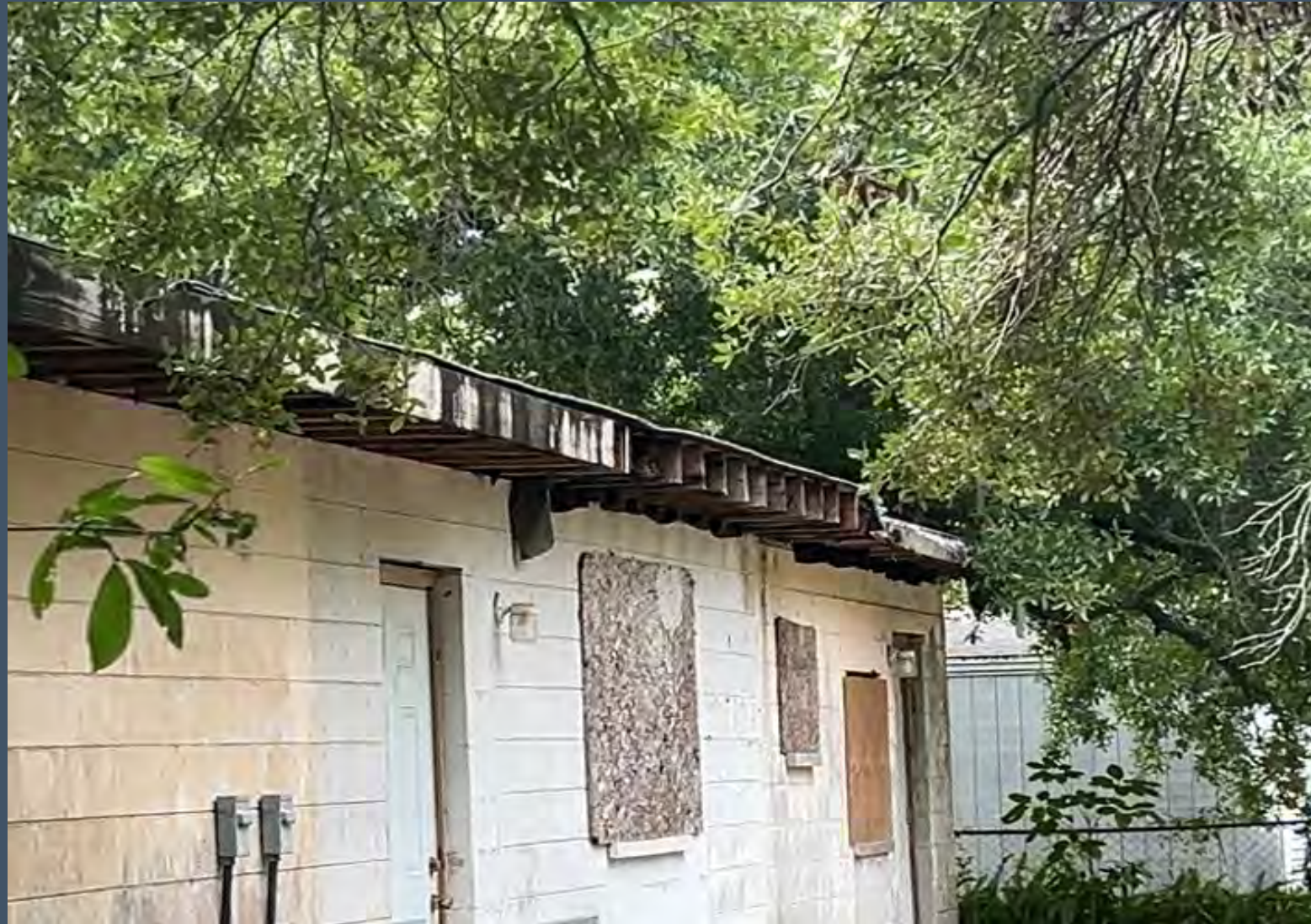
View from street of the rear roof fascia and soffit
