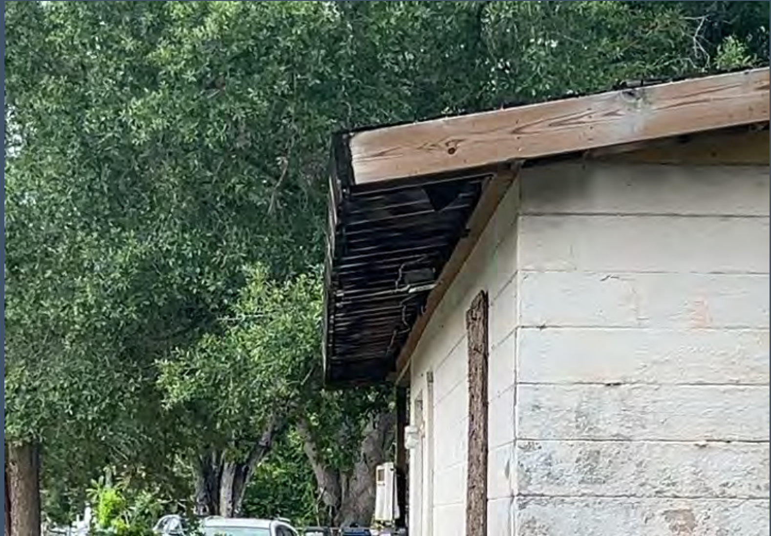
View from street of the front roof fascia and soffit
