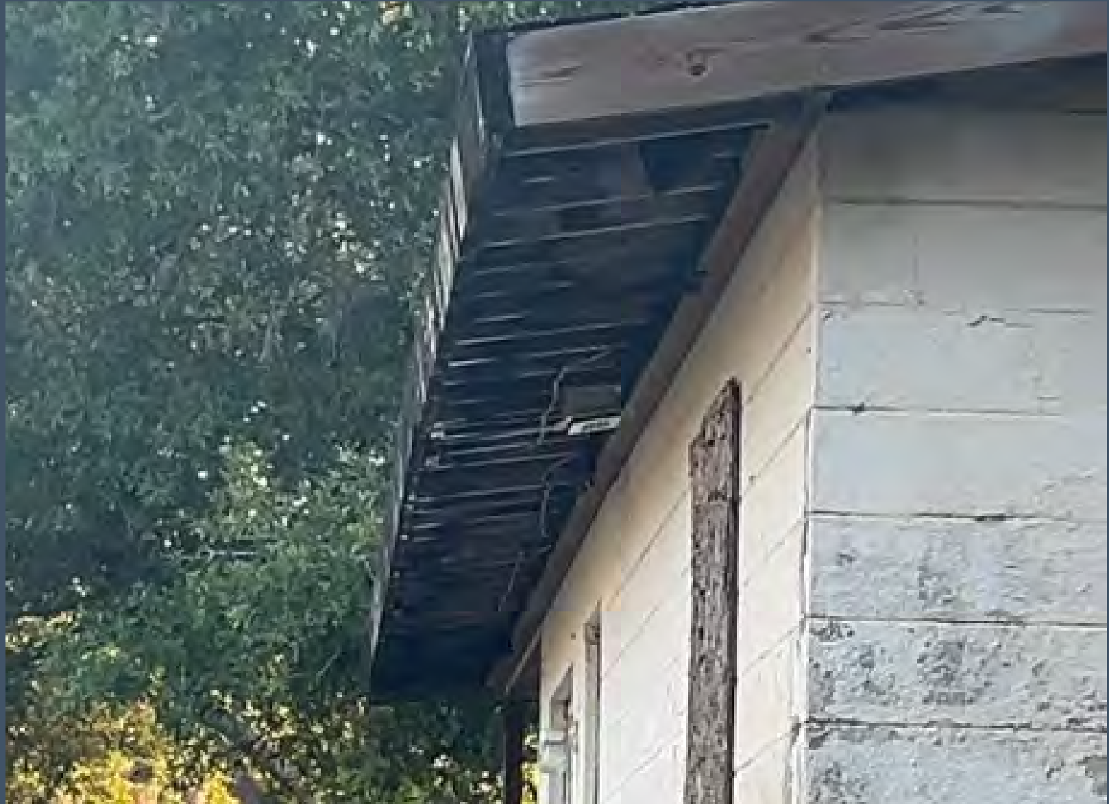
View from street of the front roof fascia/soffit
