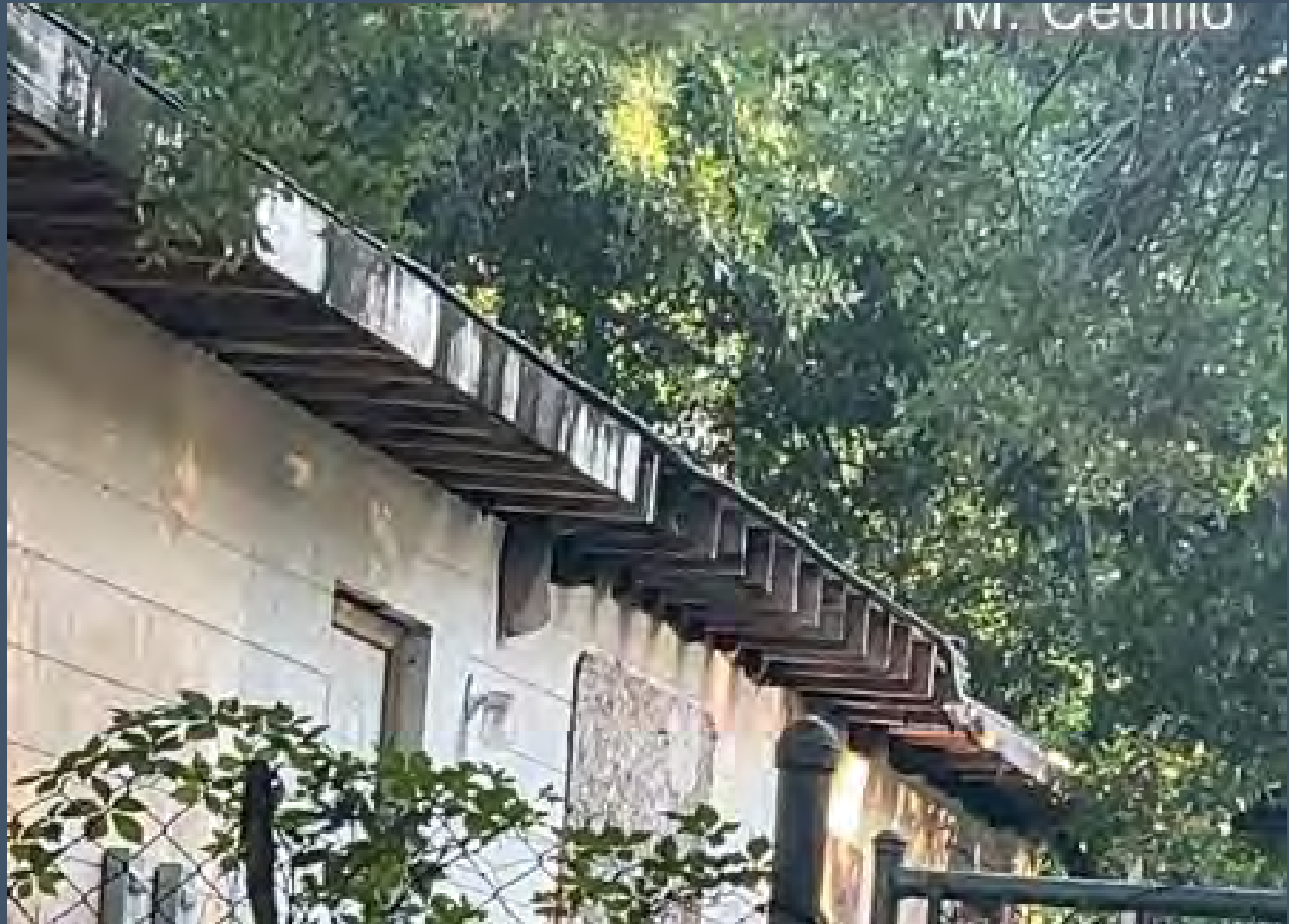
View from street of the rear roof fascia/soffit
