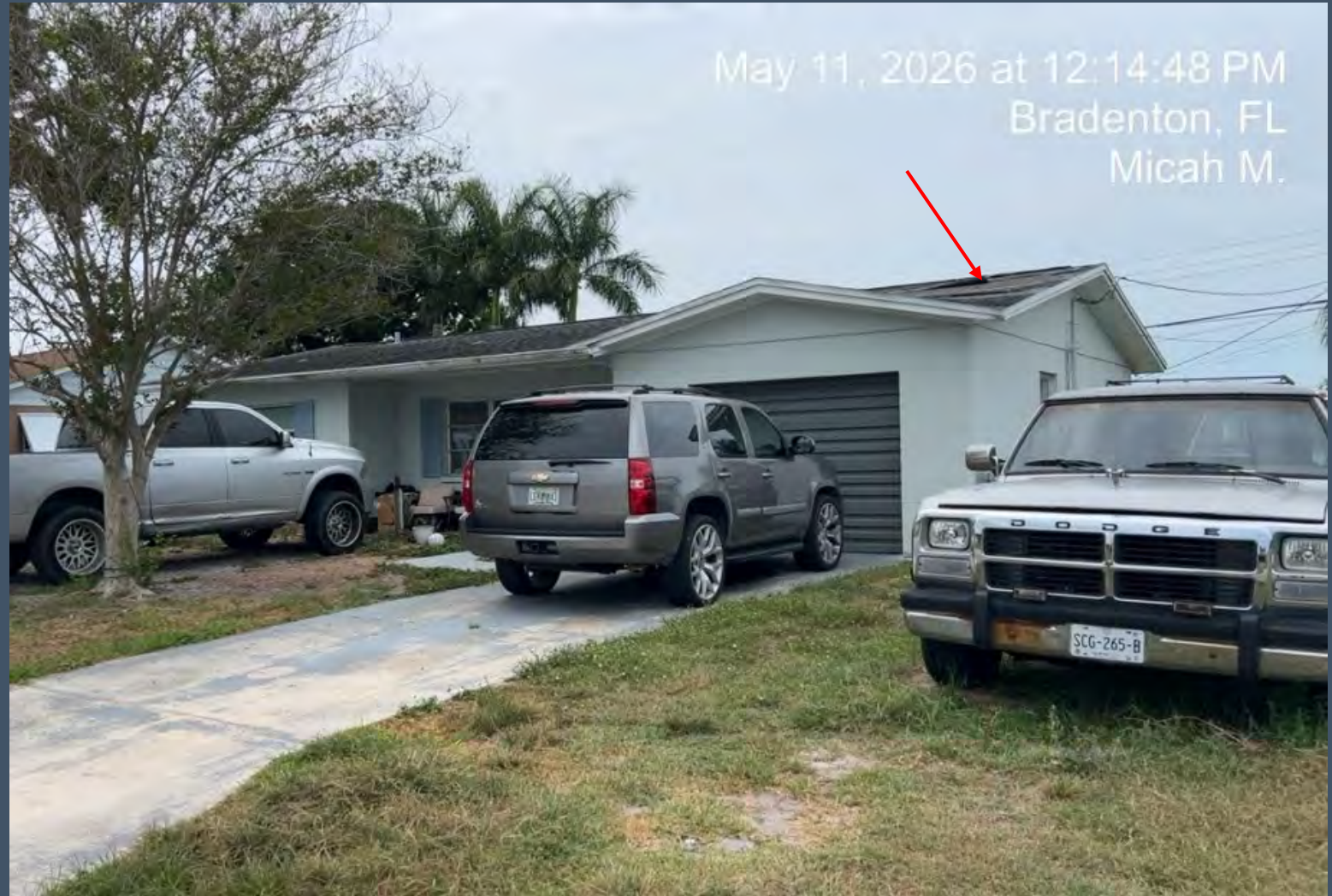
FRONT VIEW OF HOME AND THE ROOF LINE ABOVE THE GARAGE.
