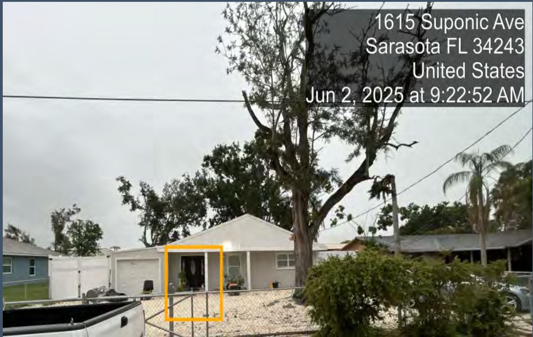
Picture of the front of the house depicting the “old door” in June 2025.
