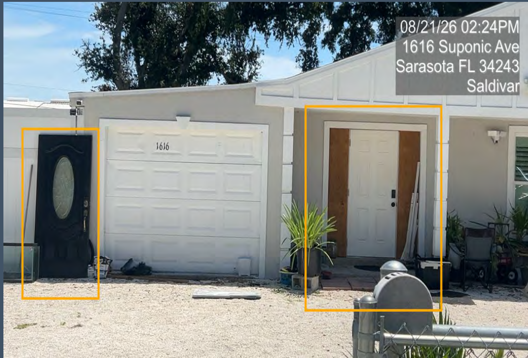
Picture depicts the front door that was removed and the new door .
