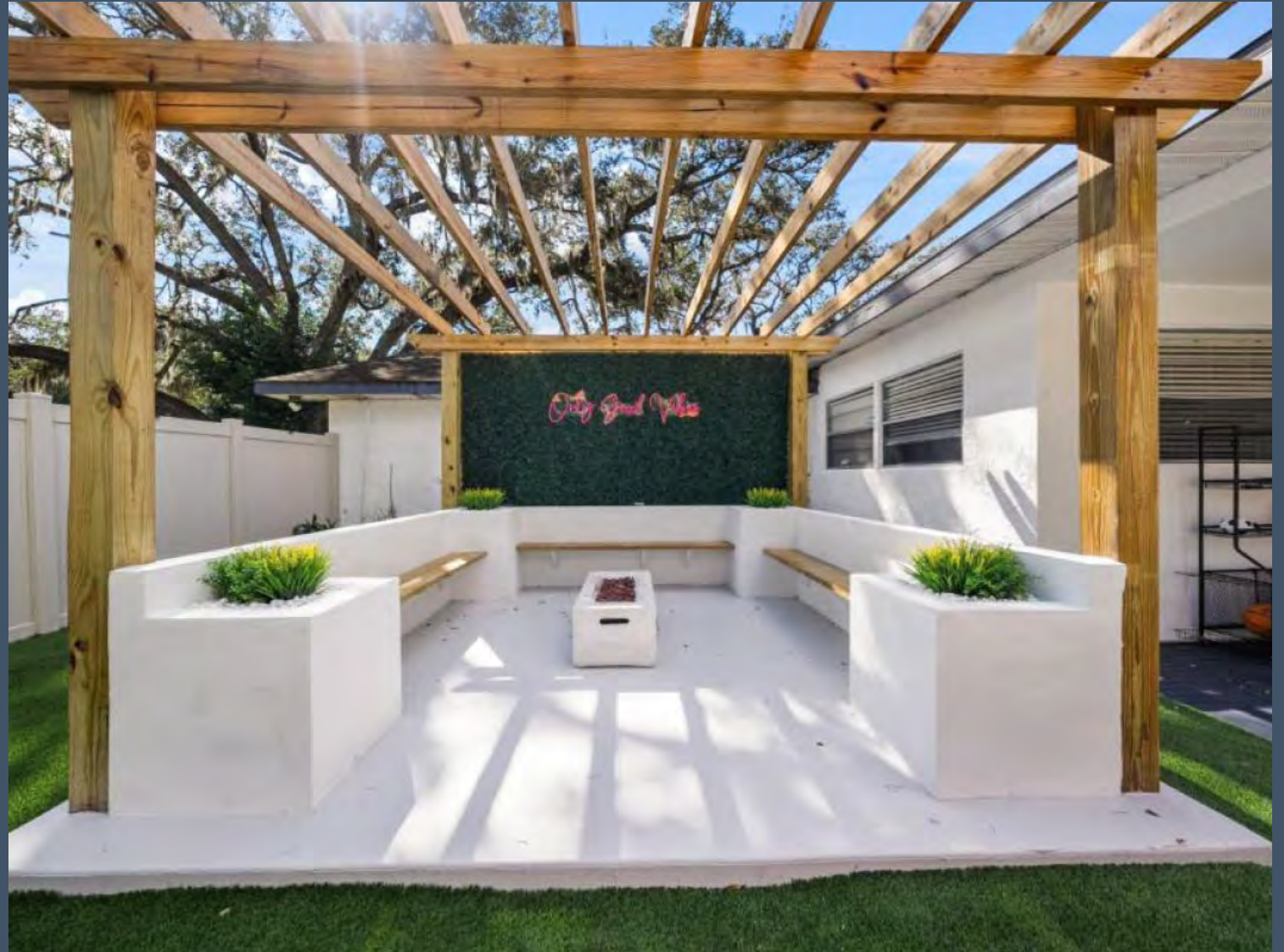
Photo from Booking.com showing the unpermitted pergola
