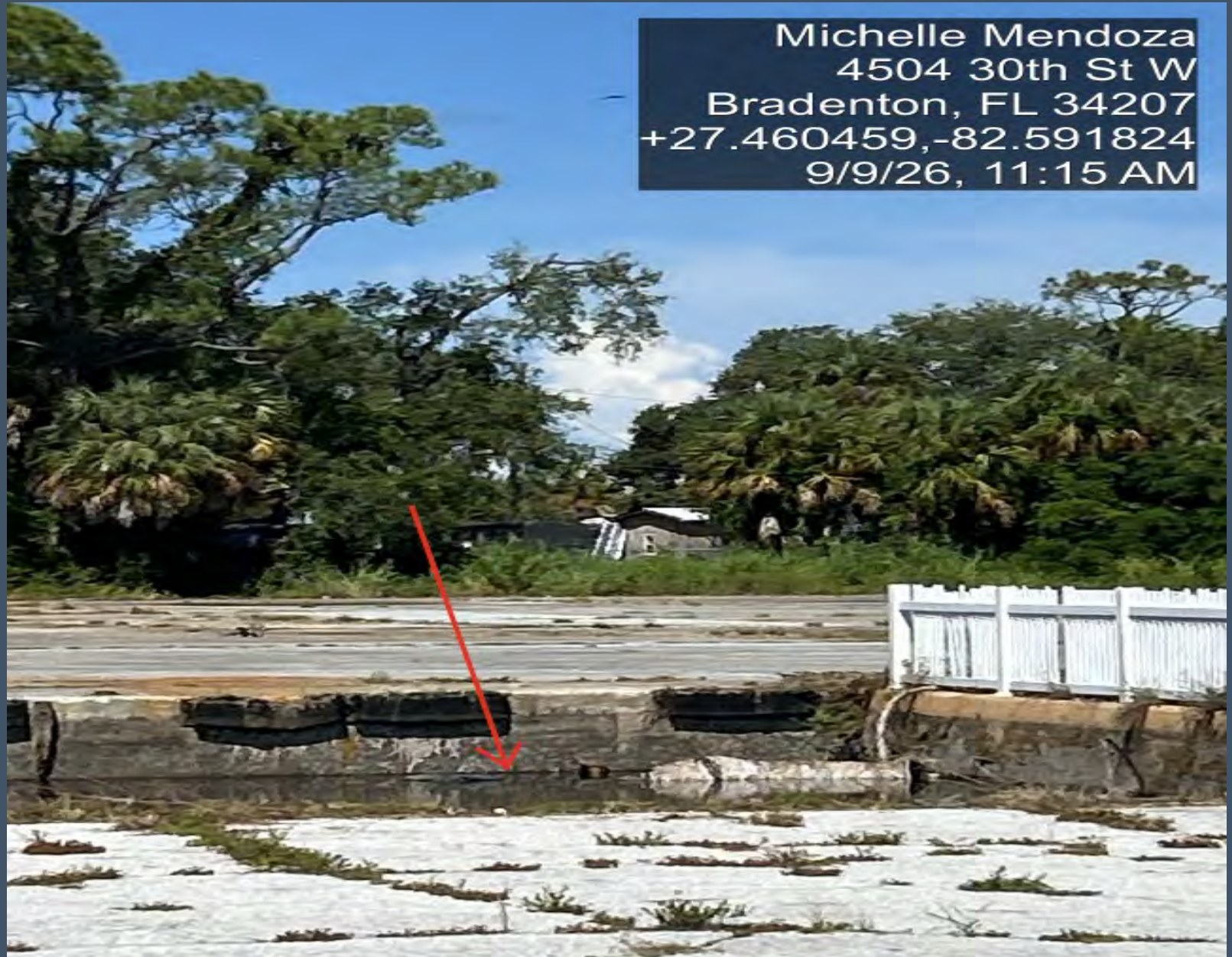
Photo of water still present in depressed loading dock.
